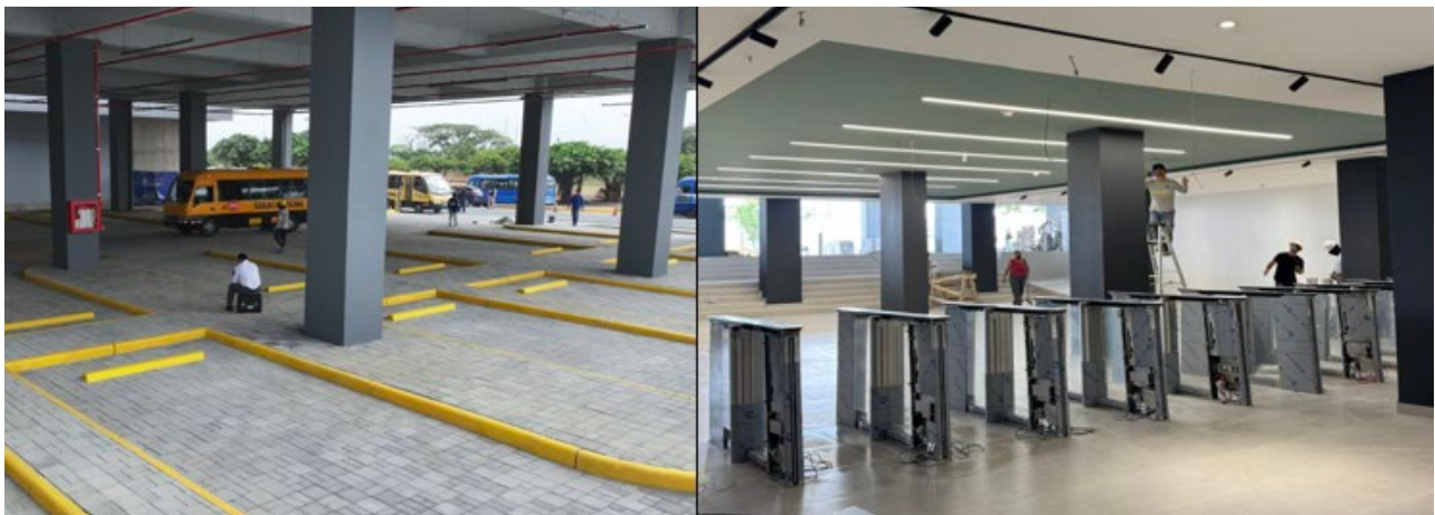
Figura 68. Terminal de Buses “Central Station” – Campus Samborondón
