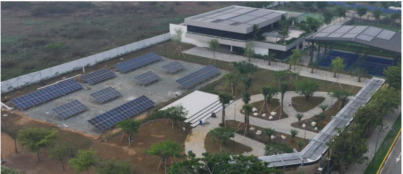
Figure 63. ECOTEC Solar Park
