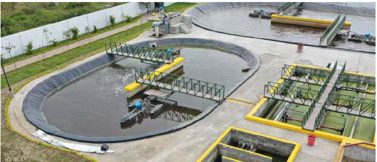
Figure 64. Wastewater Treatment Plant
