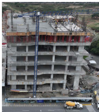
Figure 70. Construction of Building A – Samborondón Campus
