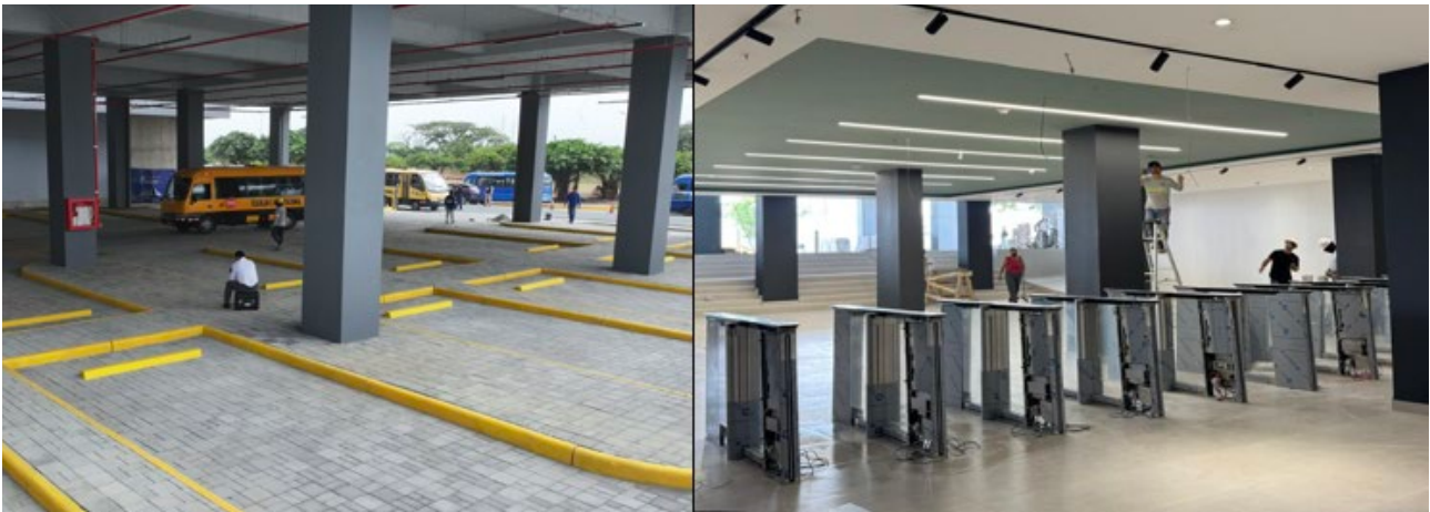
Figura 68. Terminal de Buses “Central Station” – Campus Samborondón
